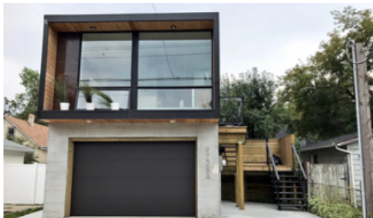
Three examples in one: a garden suite tiny home made of shipping containers. Built by Honomobo, Edmonton. Image: YEGardenSuites.com https://www.yegardensuites.com/gallery?pgid=j3stnjsa-3be-a34ed-d874-4c52-9dc2-9f0501ae2cb9
