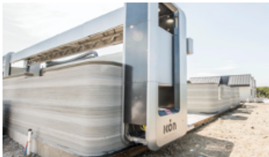
Top: 3D printed homes in Tabasco, Mexico. New Story, Icon Technologies. Image: Icon. https://www.iconbuild.com/updates/first-3d-printed-home-community
